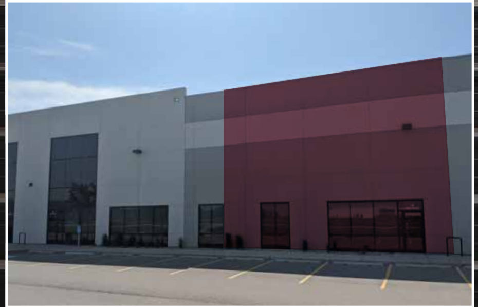
AIRPORT CROSSING WAREHOUSE 10221 15 STREET NE
